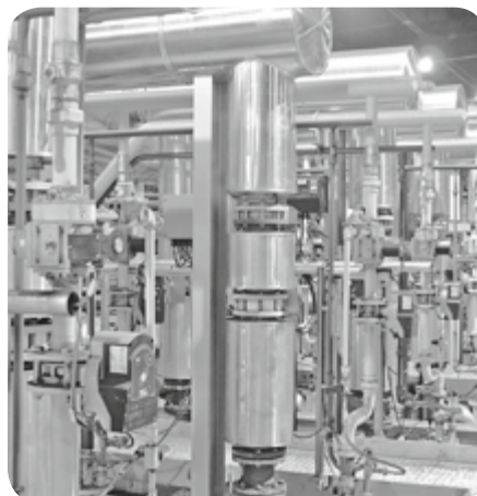
Walking beam furnace with overhead firing
